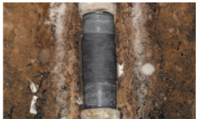
6. Pipecast after application.
