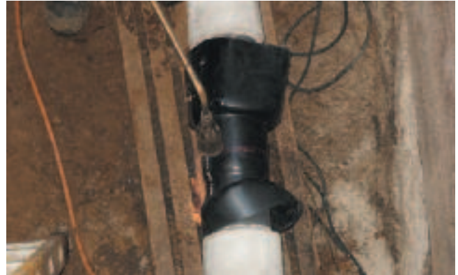
2. Installing the shrink sleeve
